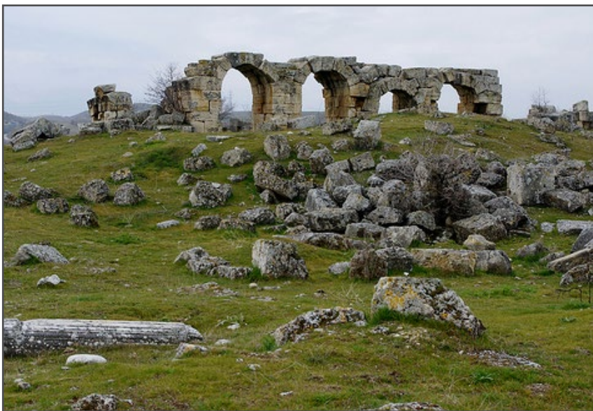
Remnants of Laodicean Aqueduct
